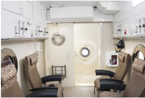
PHS 9600R Series – Dual Lock – Rectangular – 6 ATA Working Pressure – Rated for 12 patients and upto 3 attendants, installed at University of Michigan, Ann Arbor, MI
