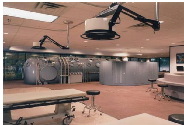
PHS 9600 Series – Dual Lock – Cylindrical – 6 ATA Working Pressure – Rated for 12 patients and upto 3 attendants, installed at Conroe Medical Center, Dallas, TX
