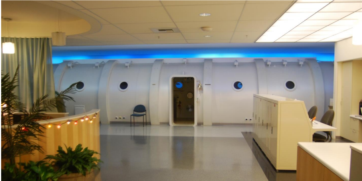
PHS 12000 Series – 3 Lock – 10 ft Diameter – 6 ATA Working Pressure - 19 to 25 patients with up to 5 attendants installed at Virginia Mason Medical Center, Seattle, WA
