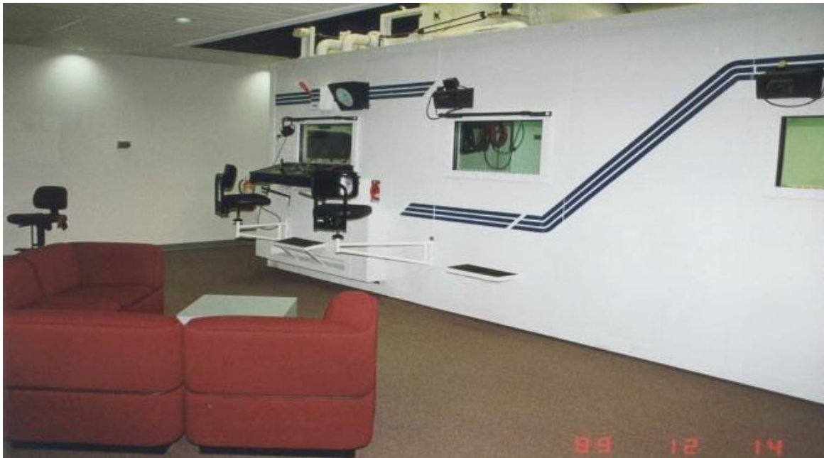
PCCI ATR-12 Series – Dual Lock – Altitude Chamber – Rated for 10 patients and upto 2 attendants, installed at University of North Dakota, ND
