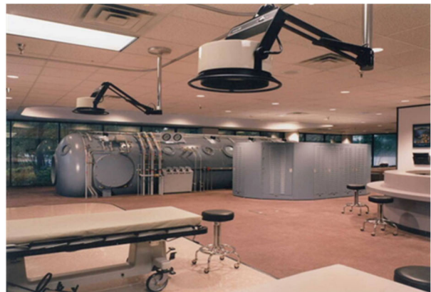
PCCI 9600 Series – Dual Lock – Cylindrical – 6 ATA Working Pressure – Rated for 12 patients and upto 3 attendants, installed at Conroe Medical Center, Dallas, TX
