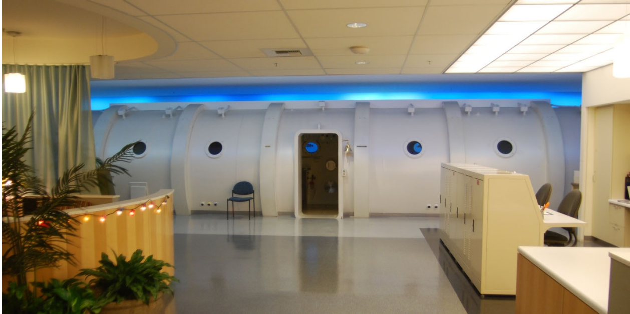
PCCI 12000 Series – 3 Lock – 10 ft Diameter – 6 ATA Working Pressure - 19 to 25 patients with up to 5 attendants installed at Virginia Mason Medical Center, Seattle, WA
